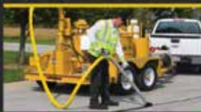
CRACK FILLING
